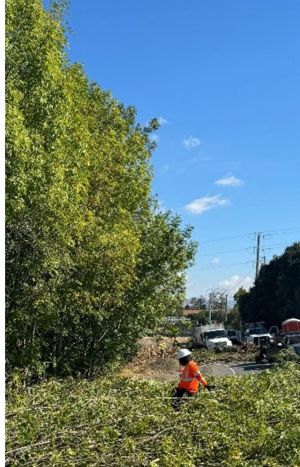
San Jose Conservation Corps workers clearing hazardous vegetation on Caltrans right-of-way.
